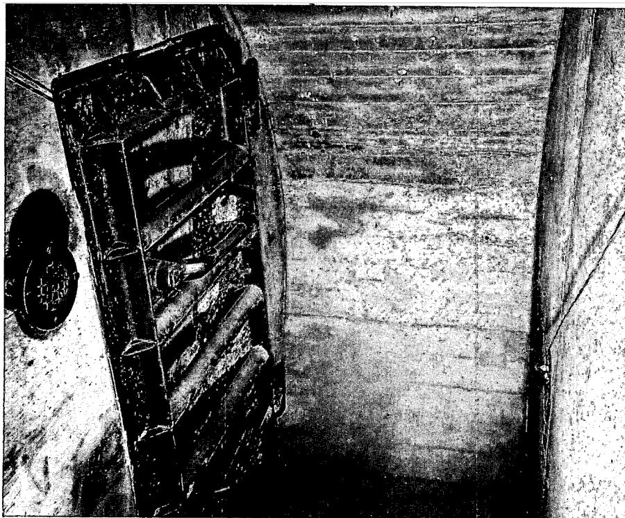
Fig. 8—Exterior view of main blast door, structure CA.
